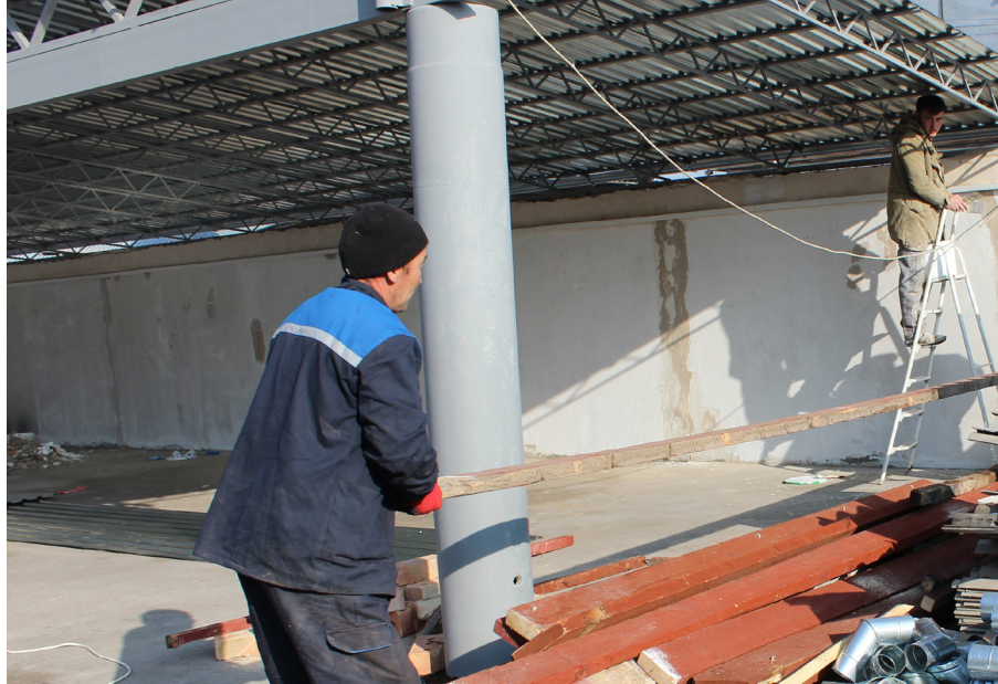
Repair and construction works in the yard of the OSCE Academy.
